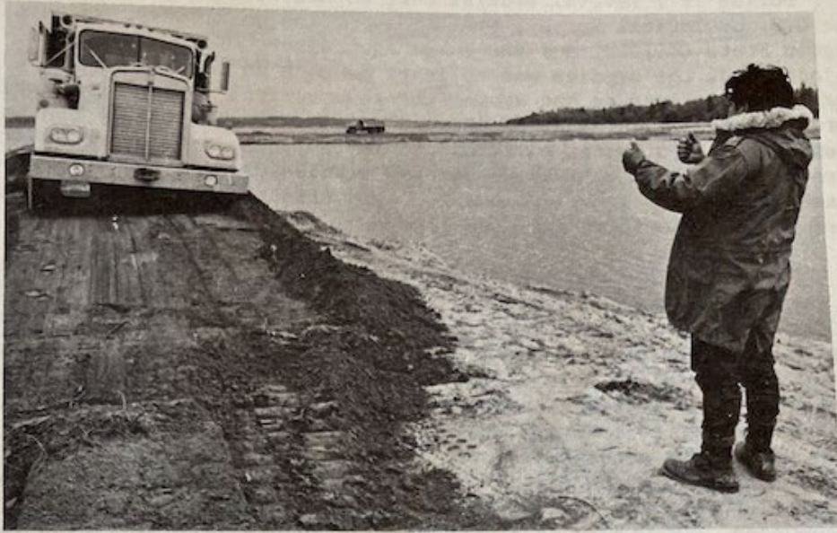
Figure 2.1 Lummi dike construction team building about 120 ft. per day between tides. Incoming tide near the end of an all-night shift. Sam Cagey directing construction traffic and spotting loads.
