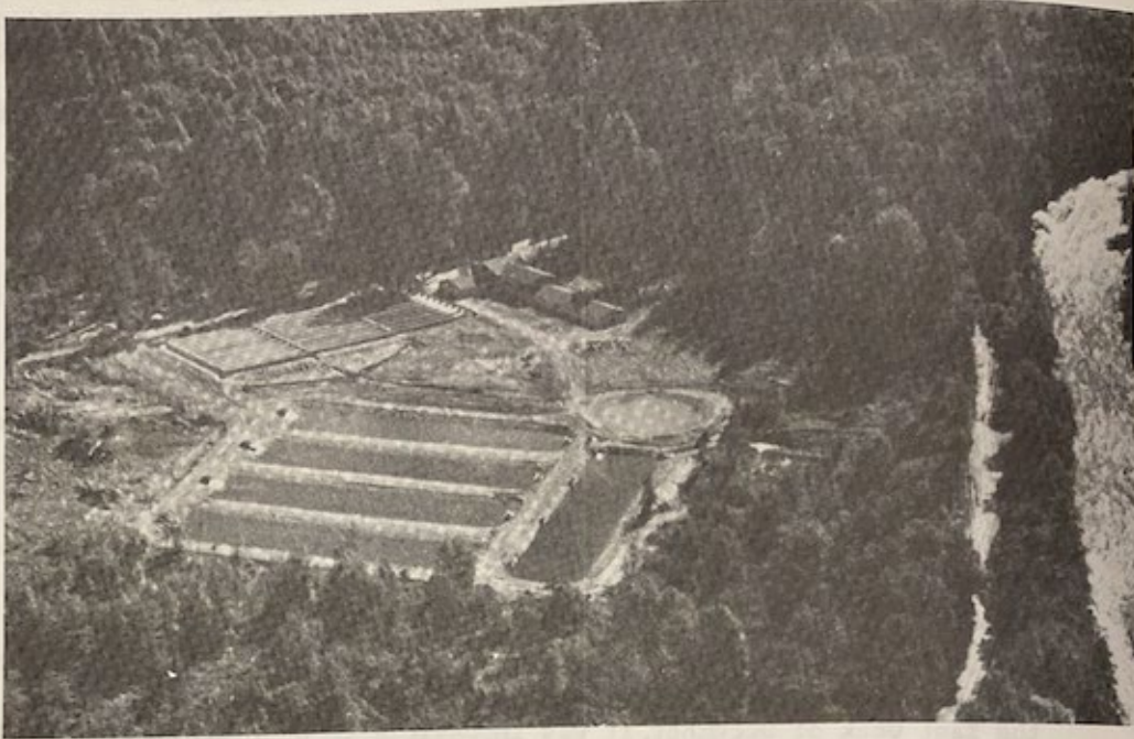
Figure 3.12 Aerial view of Lummi Fish Hatchery during late construction, Road and S.F. of Nooksack River on right.
