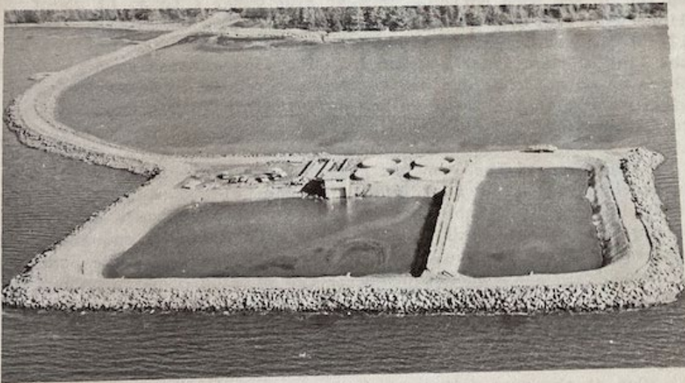
Figure 2.2 Research Ponds nearing completion. Tide fills long dirt pond at one end and standpipe regulates outflow at the other end giving 20+% exchange per day. Square tidal reservoir supplies pumphouse with sea water for six concrete ponds (see text.)
