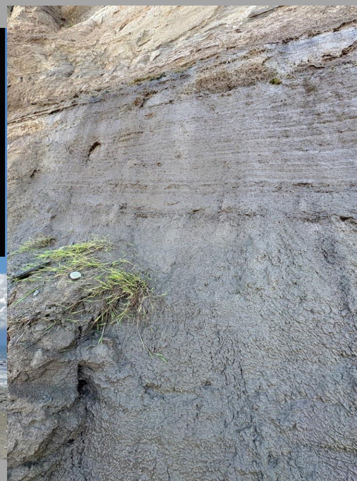
Image 2. Possible Exposed Ground Water at West Beach
